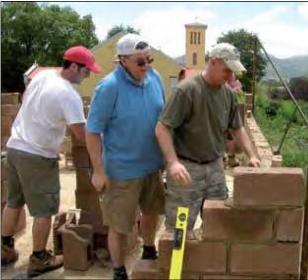
Feeding centre, under construction, in Franklin.
